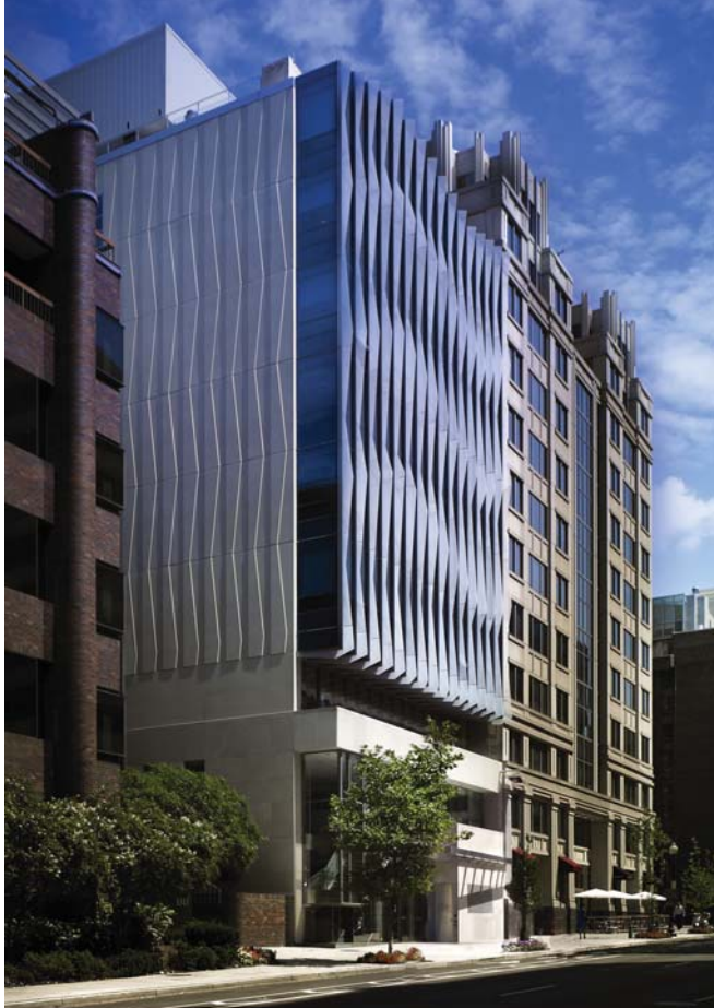
AT RISK WINDOWS ON NYU DC BUILDING
