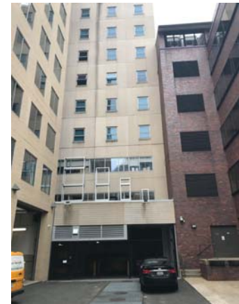
ALLEY LOOKING SOUTH
